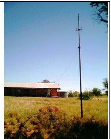
Powell Creek Overland Telegraph Station & an Oppenheimer pole
