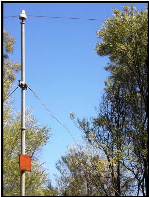
Oppenheimer telegraph pole 4E28 where the joining took place. The original pole was timber but due to the white ant problem, the timber poles were gradually replaced with Oppenheimer poles from 1873 onwards.
